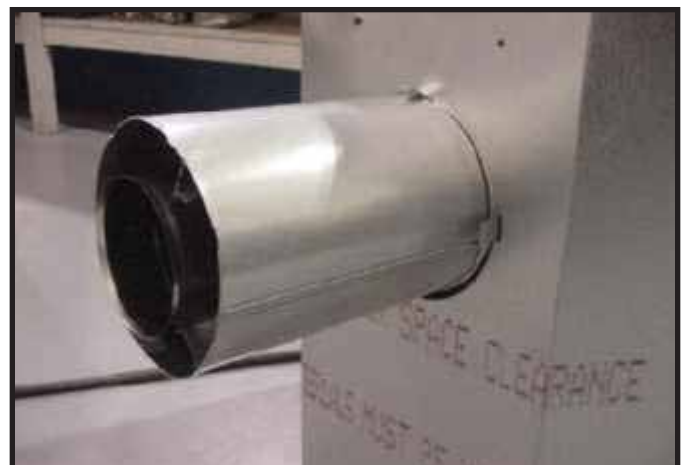
Figure 9.11 Attach the first vent section (it will snap into place). Slide the insulation gasket onto the vent section, up against the appliance and over the tabs.
